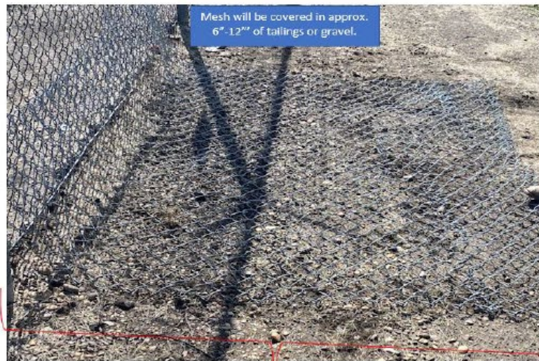
Approx. 4" coverage with gravel or asphalt tailings
