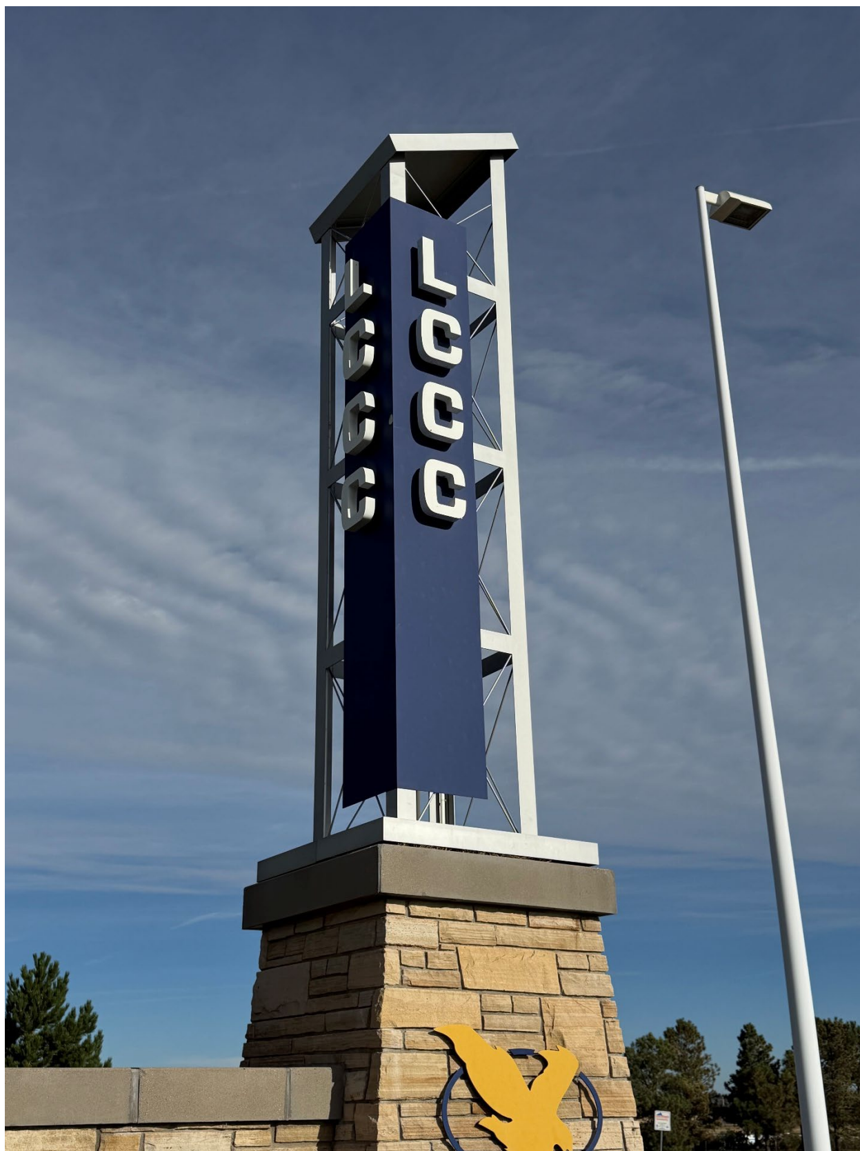
Photo 13: Spire East Entry West Side
